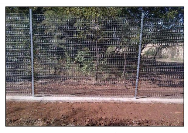
Anti-dig options are available that can be added to the fence structure namely, a concrete plinth or a mesh panel buried 16" [400mm] beneath ground level.
