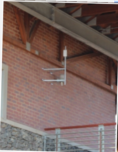
Wireless Antenna Installation
